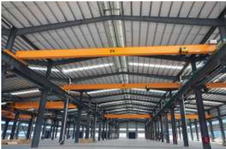
Factory building with Overhead EOT Cranes
