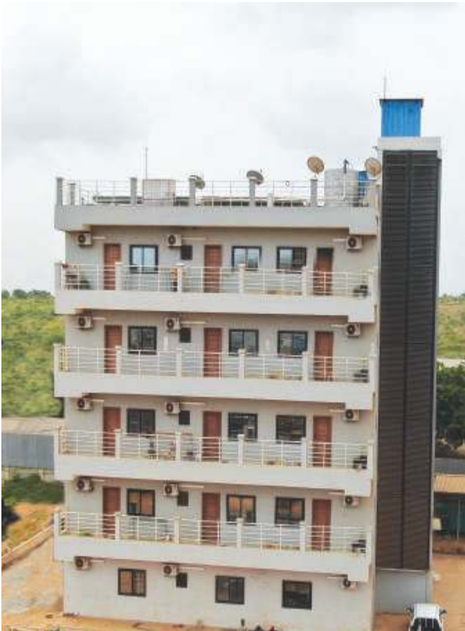
Multi-Storey Steel Building for Residential Apartment
