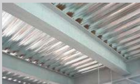
MEZZANINE FLOOR STRUCTURE
